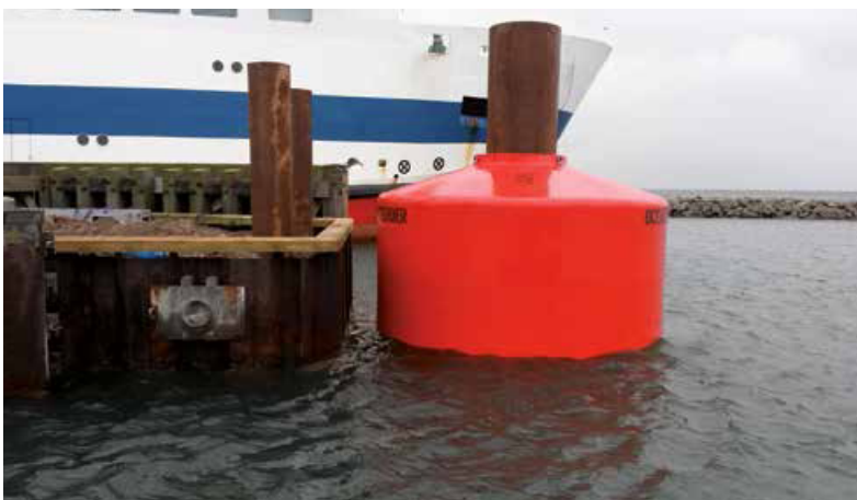
Ferry Terminal | Sejerø | Denmark
