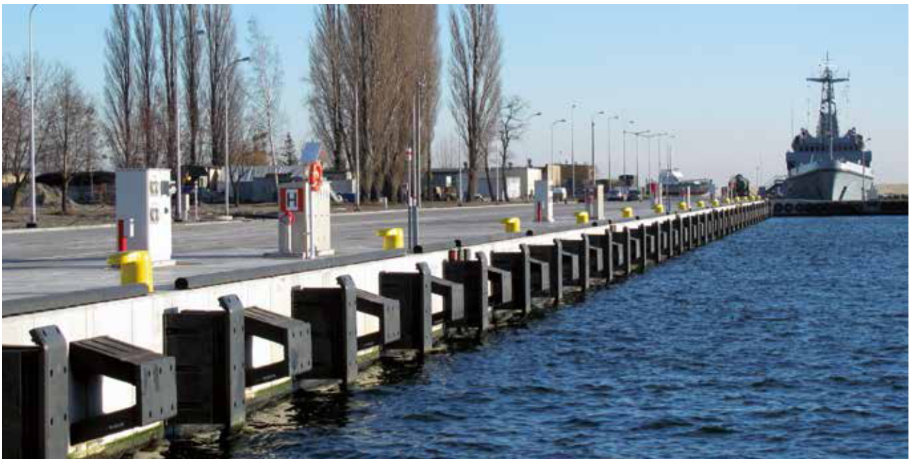
Northern Berth 16 | Port of Gdynia | Poland
