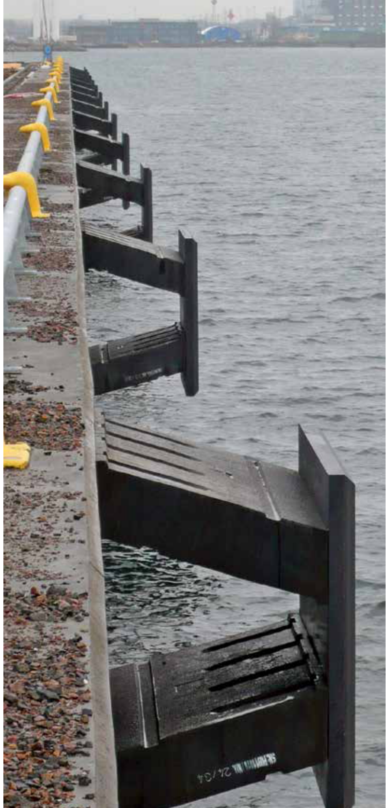
Ferry & RoRo Terminal | Malmö | Sweden
