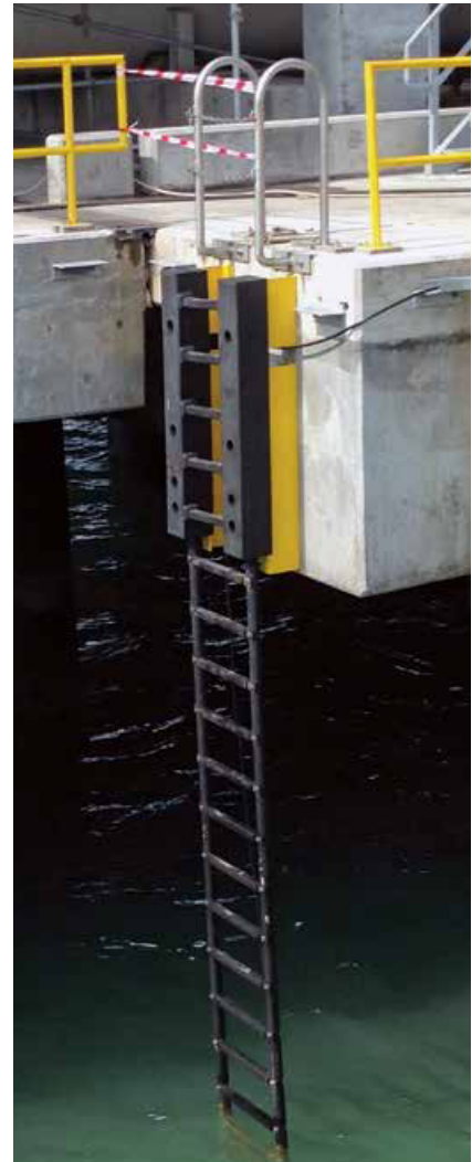
IDPT Jetty 1 | Johor | Malaysia
