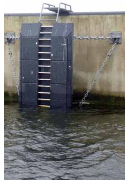
Maasvlakte II | Rotterdam | The Netherlands
