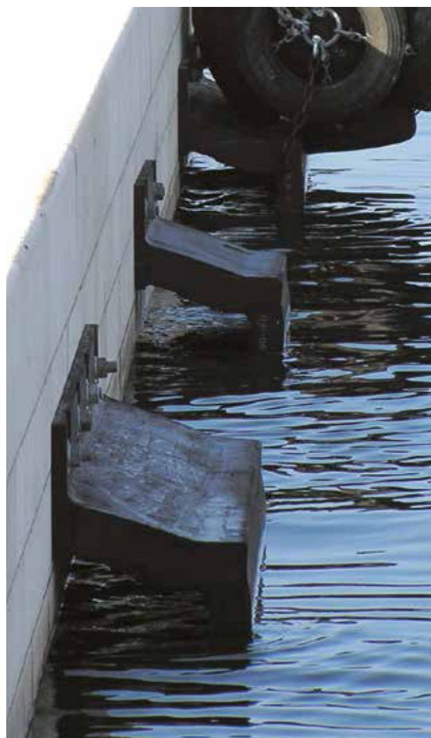
Passenger Terminal | Rijeka | Croatia
