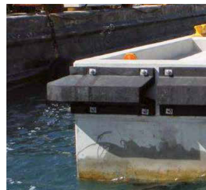
Coast Guard Terminal | Puerto Rico
