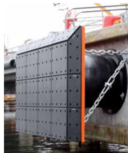
Chemical Product Jetty | Stenungsund | Sweden
