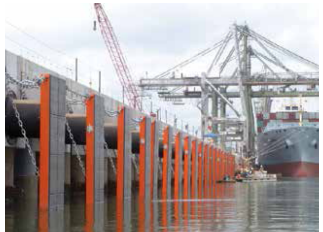
Barbours Cut Container Terminal | Houston, TX | USA
